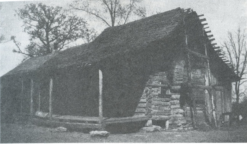
In the early years, most of Goodland's outbuildings were constructed of hand-hewn logs and rough lumber (opposite). Between 1894 and 1909 the boys lived in this log dormitory (above) (Courtesy Oklahoma Historical Society, No 19250, opposite; Taken from Sammy D. Hogue, The Goodland Indian Orphanage: A Story of Christian Missions [Goodland, Choctaw Nation: Goodland Indian Orphanage, 1940] , above).
